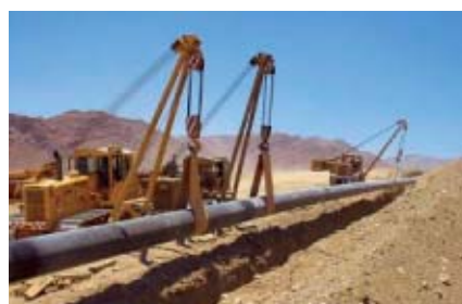
Extending Arab gas pipeline.
