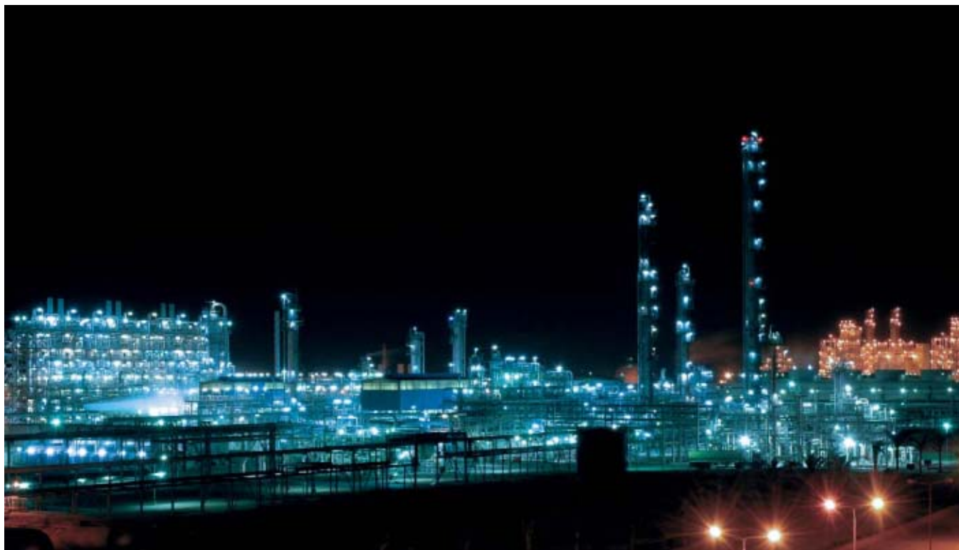
Sidpec ethylene and polyethylene plant. The company supplies all the domestic demand for polyethylene raw material.
