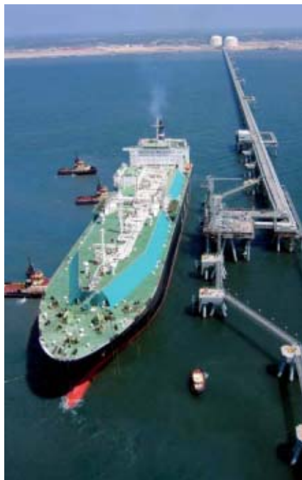
Export pipeline, Train 2, Idku.
