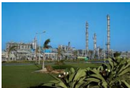
Ethylene plant overview.
