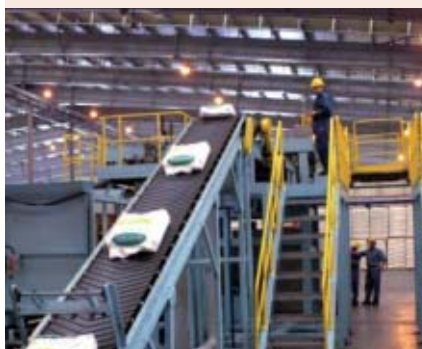
Polyethylene bagging lines.
