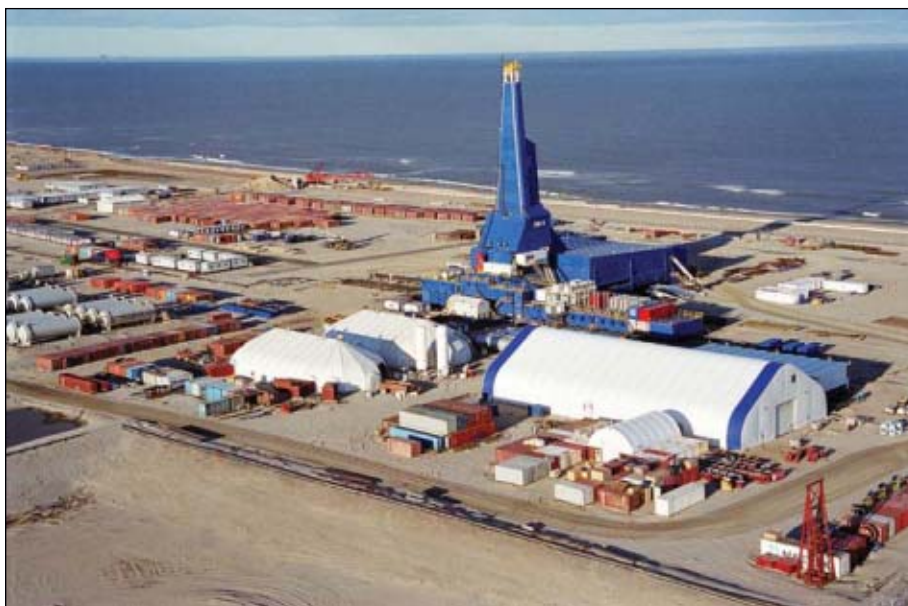
The 22-story Yastreb drilling rig, which anchors the Chayvo well site on Sakhalin's northeast coast, was designed to drill extra-long extended-reach wells nearly 11 km offshore. Photo from ExxonMobil.
